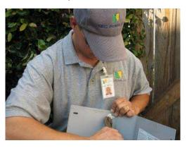
Remove the cycling device from the A/C unit and seal <sup>3</sup>/<sub>4</sub>" hole seal to plug opening.
