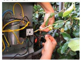
Splice into the white thermostat wire with the open yellow wire and cap it.
