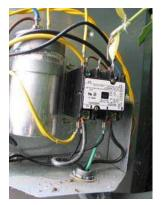
In order for the cycling device to work properly, you will need to tap into power to power the cycling device and connect cycling device wires into the thermostat and control wires. These are the steps you will follow:
