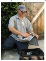
Use a cordless electric drill to drill a 3/8-inch pilot hole through the A/C case. Next, use a Greenlee 1-1/8 inch chassis punch or equal and punch the required hole.
