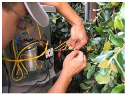
Disconnect the two yellow wires from the thermostat control wires and rewire them to original condition.
