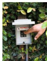
Provide proper weatherproofing at all areas affected by mounting and cable connections so that the completed installation is rain tight.
