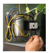
Disconnect the two power wires (black) from the contactor.
