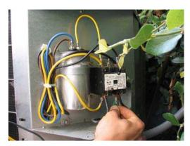
Connect the female disconnects on the black cycling device wires to the open copper tabs, on the load side.
